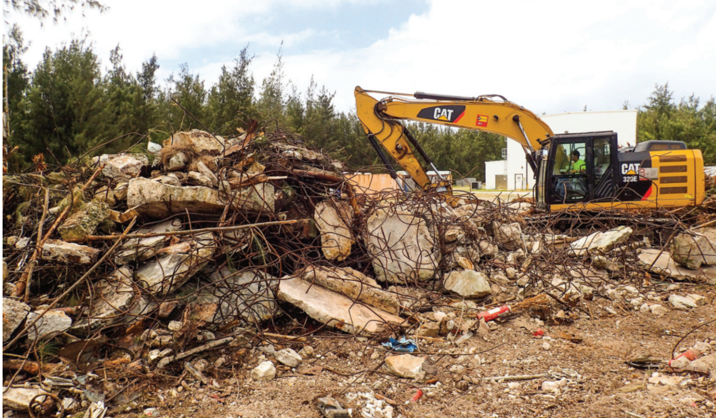
Trees, shrubs, and surface debris near or within solid waste areas were cleared using an excavator. PHOTO COURTESY BRICE ENVIRONMENTAL
