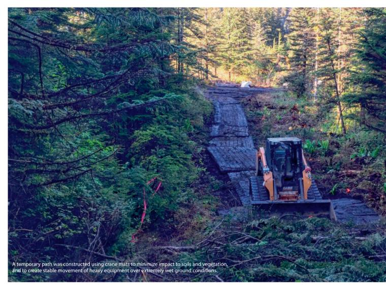
The use of lightweight crane mats to construct a temporary path for heavy equipment was proposed. Though still not ideal, the Forest Service and the U.S. Fish & Wildlife Service weighed all options and ultimately approved this solution. Mats were inspected to ensure no transfer of invasive species and the Forest Service walked the proposed pathway for mat placement to safeguard historical sites. With mats in place, Phase One moved forward.
